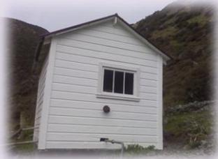
The work on repairing the historic pump house continues at a slow but steady pace. The replacement window has been installed and primed, with only a couple of top coats now needed to complete it. Our project manager, Richard Nester, has arranged with our joiners, Cheriton Classique, for the construction and installation of a new door. Our thanks go to Cheriton Classique for generously donating their time for this part of the project.
